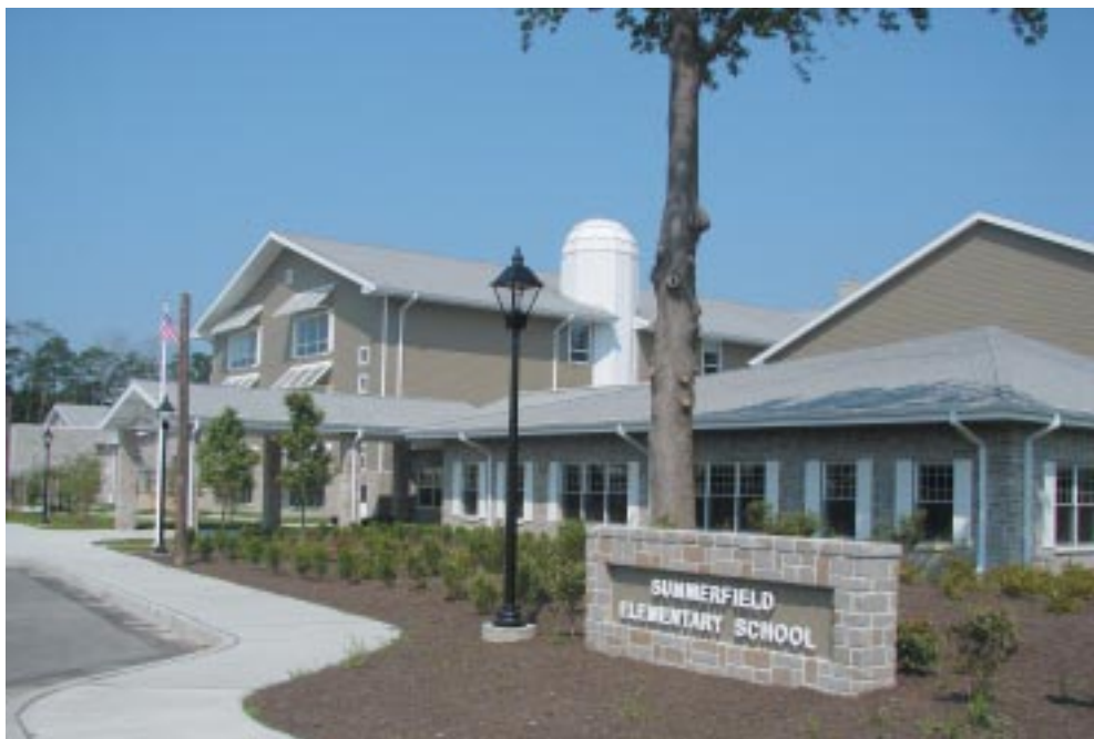
Summerfield Elementary School opened in spring 2006. The facility’s designers expect the school to earn LEED Gold.
